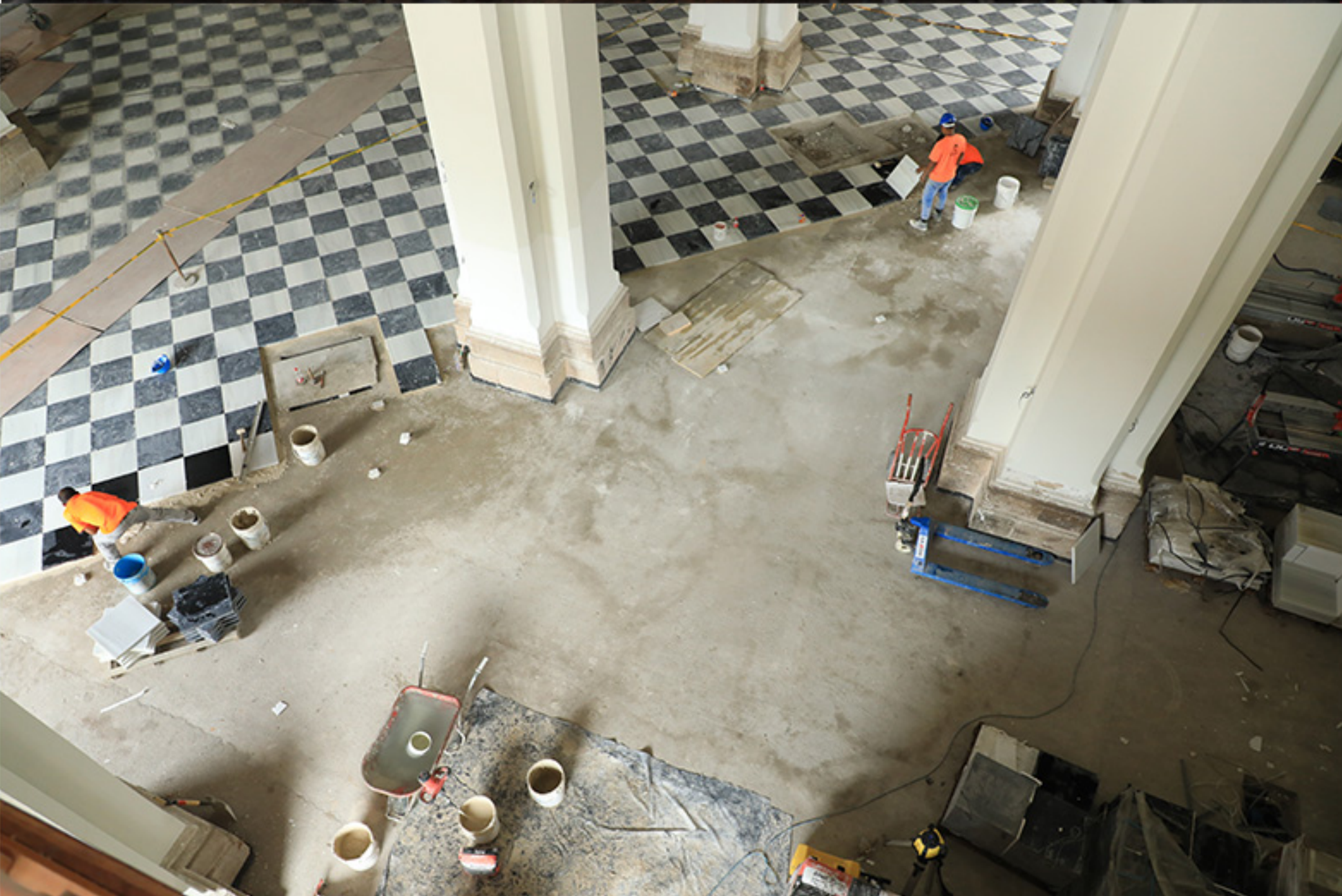
The flooring from the 1600s was removed, revealing some surprises including skeletons!
