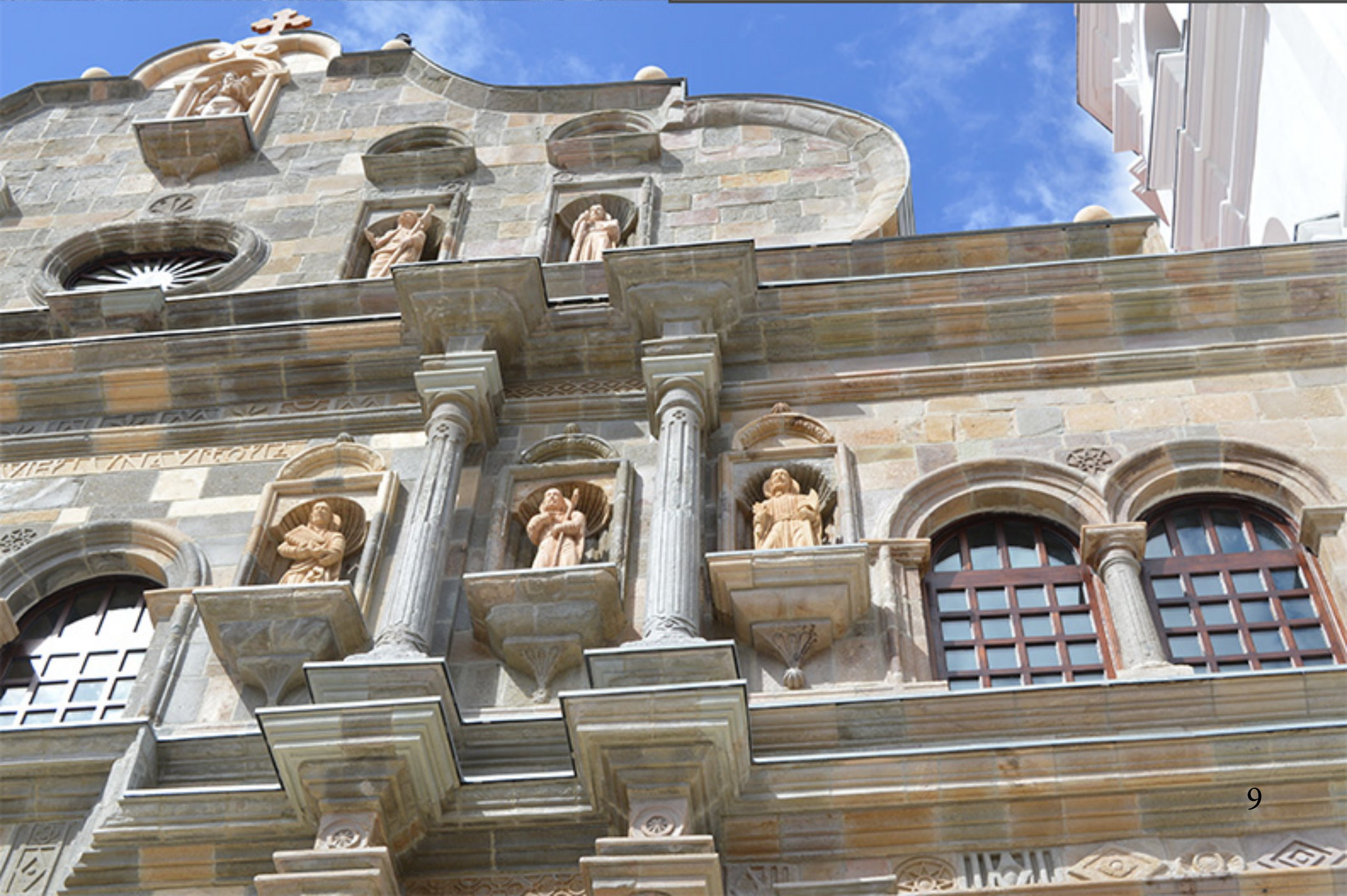
The exterior of the Catedral Basilica Santa Maria la Antigua also received a facelift.
